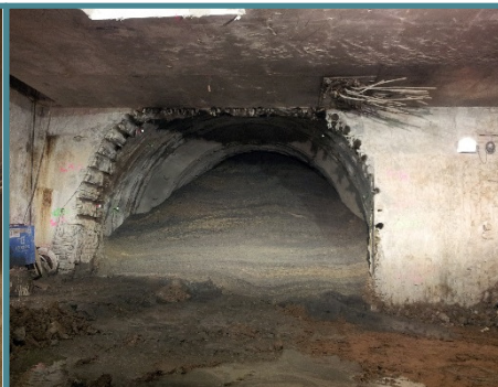
Tunnel collapse and in-filling, leading to flooding of access shaft (Poland)
