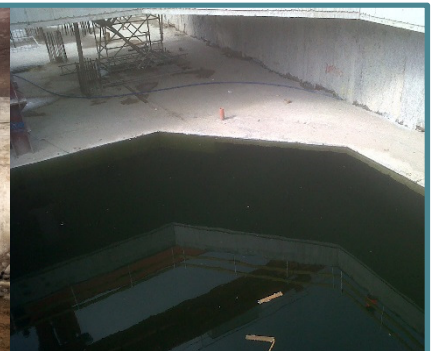
Tunnel collapse and in-filling, leading to flooding of access shaft (Poland)
