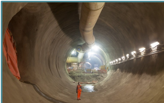
Crossrail Farringdon Station Platform Tunnels (UK)
